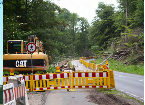
PICTURED: BARRICADE LIGHT IN USE
